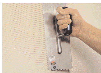
...the KÖSTER AMS 3 Special Plaster is applied uniformly thin...
