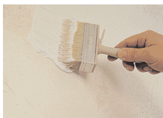
... the KÖSTER AMS 2 Liquid Film is applied. After 1 hour curing time...
